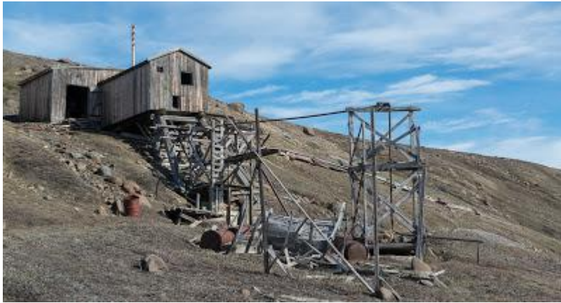
Old mining shaft at Qullissat
